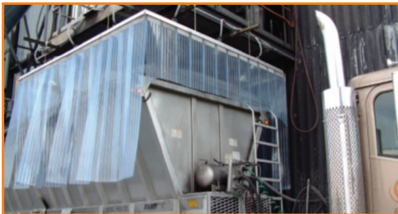
Figure 23: Covering loading and unloading areas with flexible plastic sheets (with hopper)
