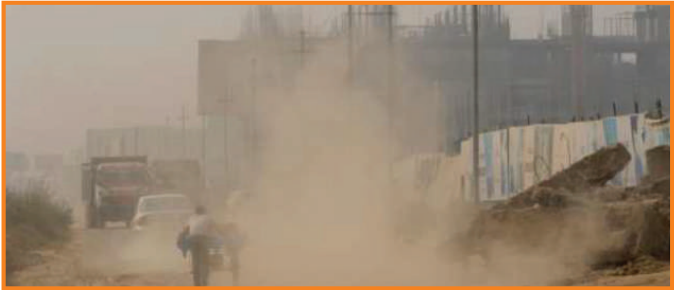
Figure 19: Unpaved Road and Construction dust
