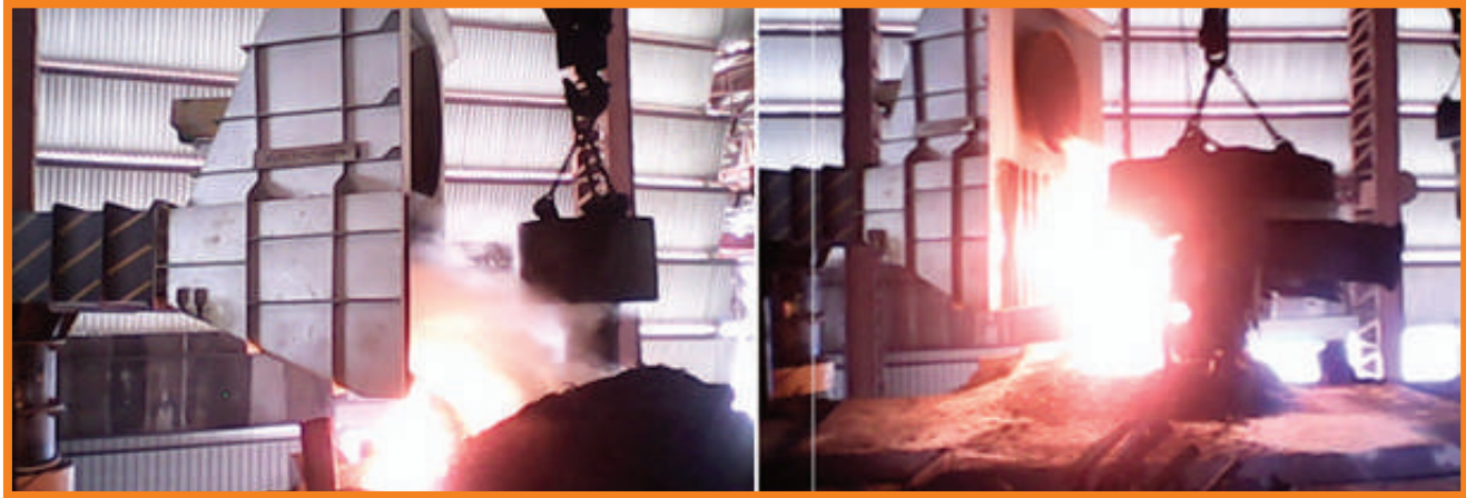
Figure 18: Sideways collection of fumes from melting and casting operation
